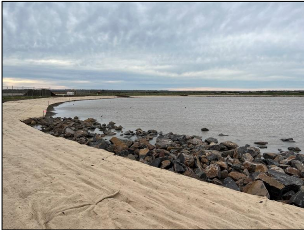
Plate 1. Jute matting and rock piles installed around the edge of the created wetland (Ecology and Heritage Partners 15/08/2025)
